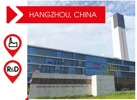
TCAC - PRODUCTION FACILITIES
