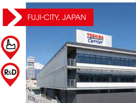
TCC - PRODUCTION FACILITIES and TCC - ENGINEERING CENTRE
