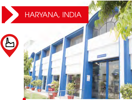
TCAI - PRODUCTION FACILITIES
