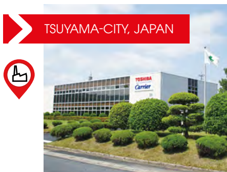
TCC - PRODUCTION FACILITIES
