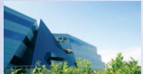
Montilla Cordoba Spain Industrial site for Air-Air units
